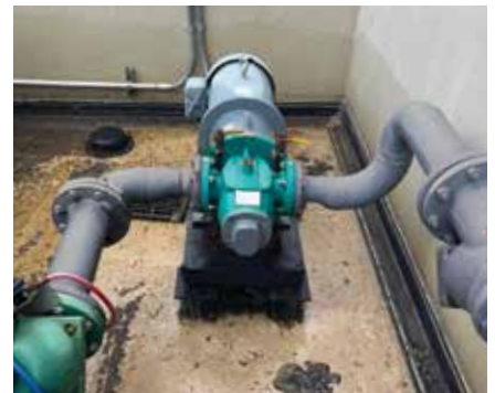
NOTOS® Multiple Screw Pump - in a mineral oil transfer application between tanks.
