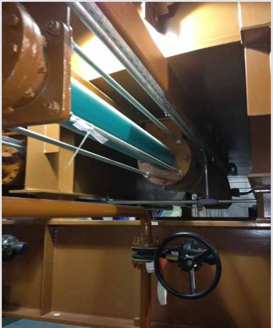
NETZSCH engineers designed the NEMO progressing cavity pumps with a customized hopper that allowed the customer to use the existing silo bolt pattern, simplifying installation
