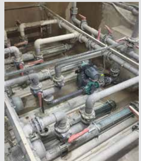
The NETZSCH TORNADO® T2 Rotary Lobe Pump requires a relatively small footprint and provides ease of maintenance.
