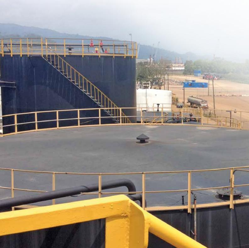
Tank farms form the backbone of many industries, especially in the oil and fuel markets, as storage tanks or intermediate storage facilities. However, these media have a higher viscosity that makes the tank stripping, i.e. the pumping-out of the residues, difficult. Remaining substances reduce the useable tank volume. To secure the maximum available storage space, more companies in these markets have recognized the value of using positive displacement pumps from NETZSCH.
