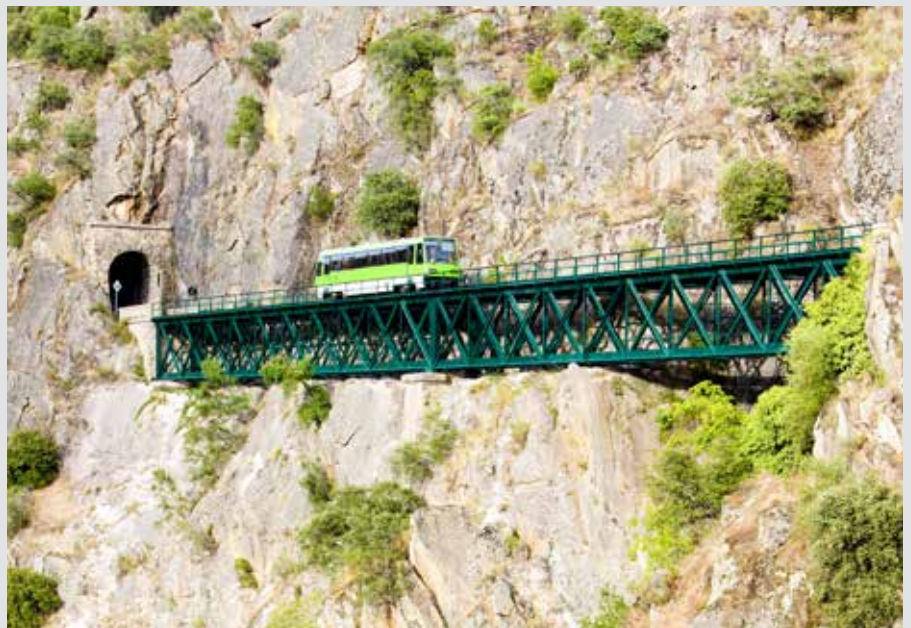
Viaduct near Tua, Douro Valley, Portugal
