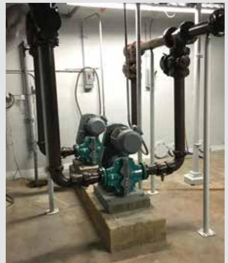
The NETZSCH TORNADO® T2 Rotary Lobe Pumps in the Plainwell Water Renewal facility requires only a small footprint while providing easy access for maintenance.
