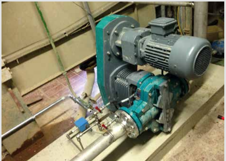
The NETZSCH TORNADO® T2 Rotary Lobe Pump requires a relatively small footprint and provides ease of maintenance.
