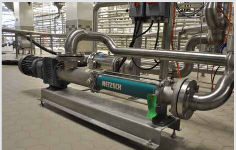
Over the course of brewing, the yeast involved in brewing can quadruple in quantity. This spent yeast is removed from the liquid through filtering, suctioning or settling. (pumps 4 & 5).
