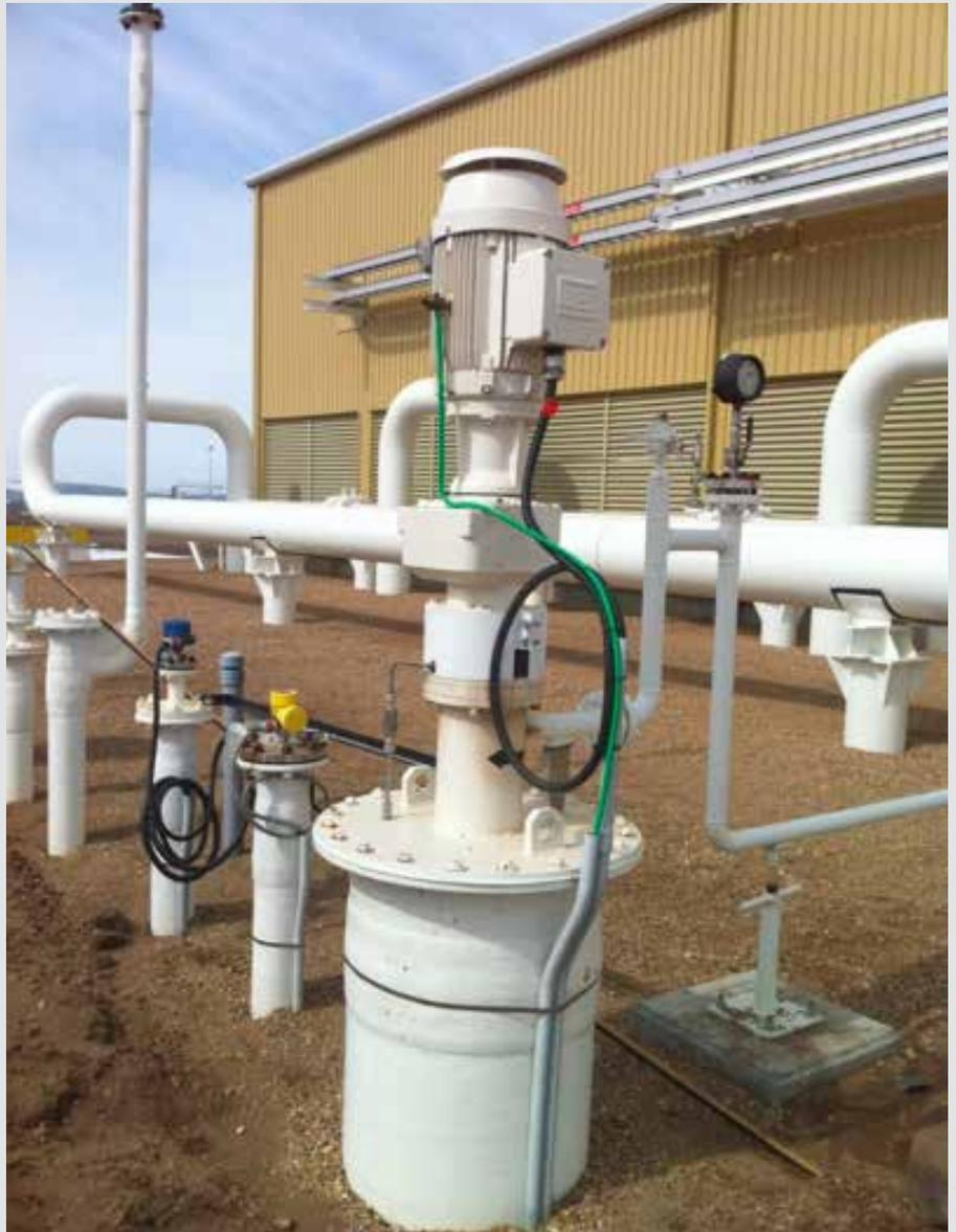
A need to reduce maintenance and simplify the transfer of oil from an underground tank back into the pipeline required NETZSCH to design and build a custom, 10-stage vertical progressing cavity sump pump to satisfy customer requirements.
