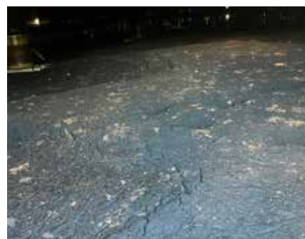
Sludge collected at the bottom of tanks
