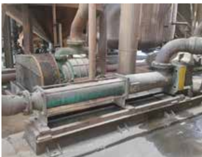
NEMO® SY pump transfers lime milk
