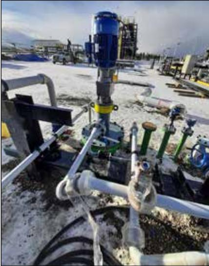
NETZSCH NEMO® BT is installed on top of the drum which is below grade.
