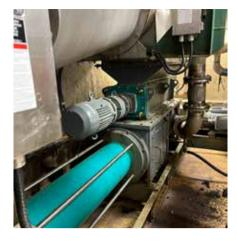
B.Max® pump housing, allows for comprehensive maintenance of the robust Z-joint and cutting device replacement without the need to remove the entire grinder. This is a significant advantage given the challenges of performing maintenance in the cramped space where the system is located.
