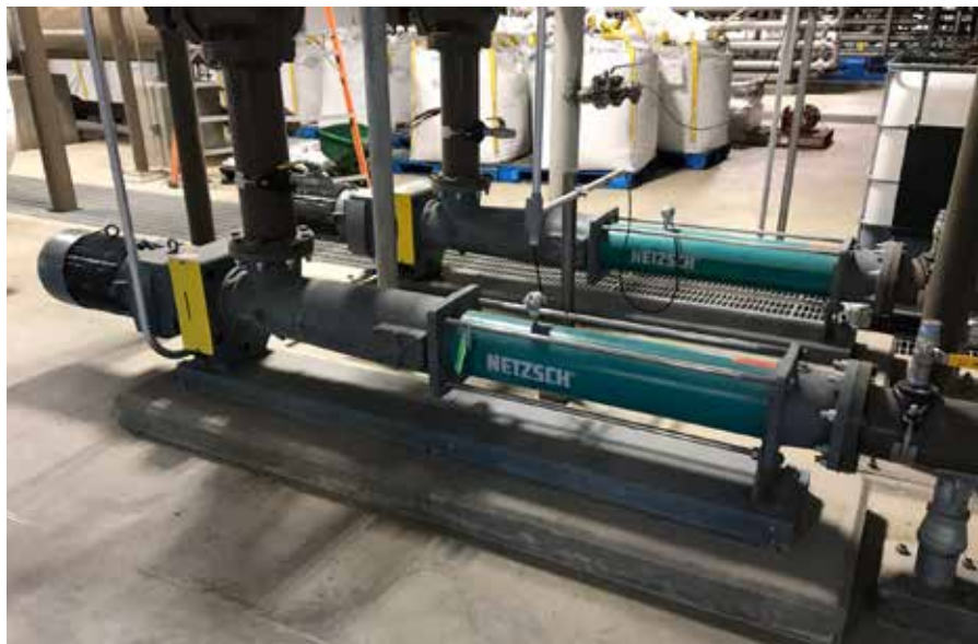
NETZSCH NEMO® 090 BY pumps in the Boiler Building provide a feed to the Struvite production.
