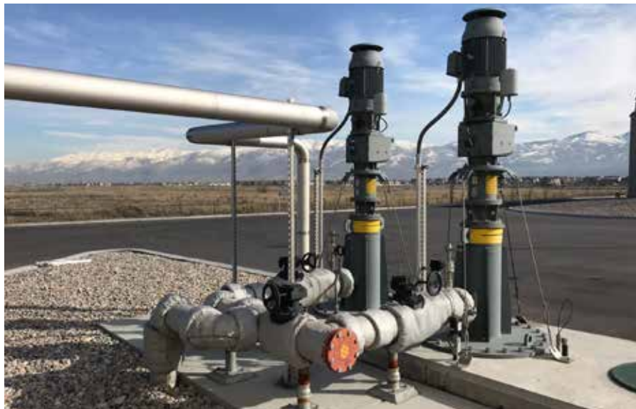
NETZSCH NEMO® BT pumps for hydrolysis feed at liquid wasterreceiving building (liquids, de-packaged waste from dog food, food products, fruits, grocery waste, and produce.
