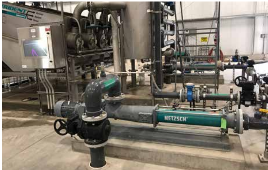
NETZSCH NEMO® FSIP® pumps in the chemical recovery building pumping post struvite production to water removal
