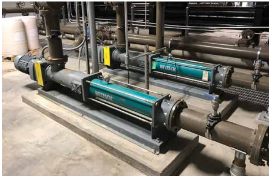
NETZSCH NEMO® 090 BY pumps in the Boiler Building transfer hydrolized food waste with extremely low pH product with 5% solids.
