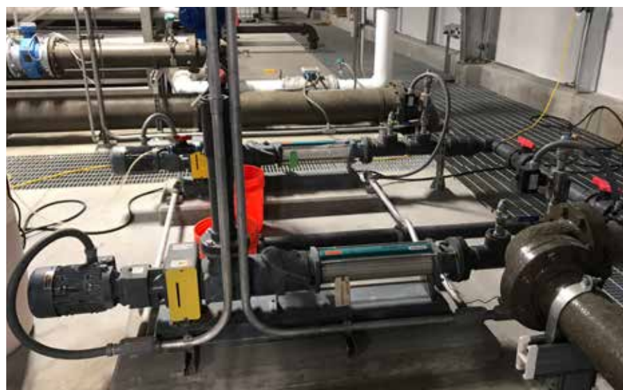
NETZSCH NEMO® FSIP® pumps in the boiler building to pump grease trap waste from restaurants and bacon grease from local bacon manufacturer to convey product to the digesters.
