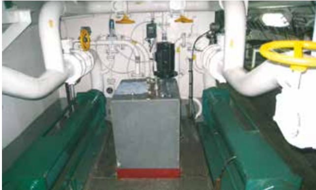
NEMO® pumps to transfer kaolin on board
