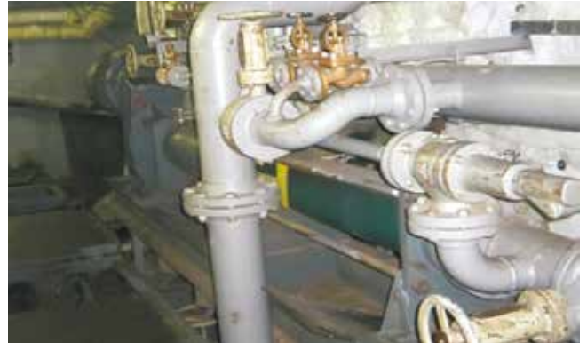
NEMO® pump to transfer sludge
