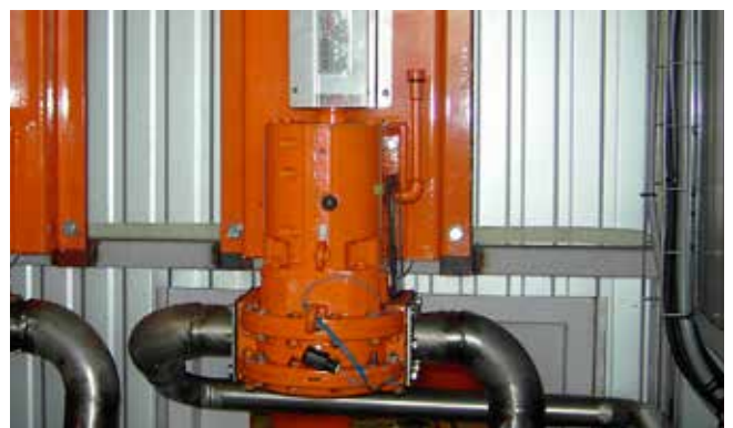
TORNADO® pump for sewage water
