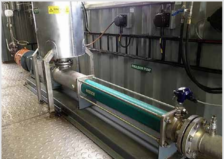
The NETZSCH NEMO progressing cavity pump seen here is dramatically improving life-cycle costs and uptime for a customer's explosive emulsion manufacturing process.
