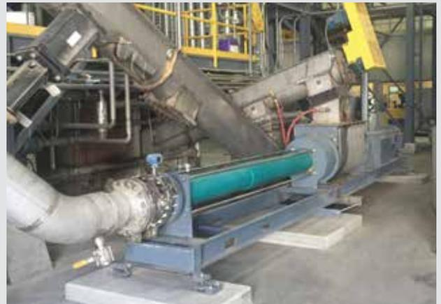
The NETZSCH NEMO® SF Progressing Cavity Pump in the Pacific Ethanol facility has a customized system to move wet cake.
