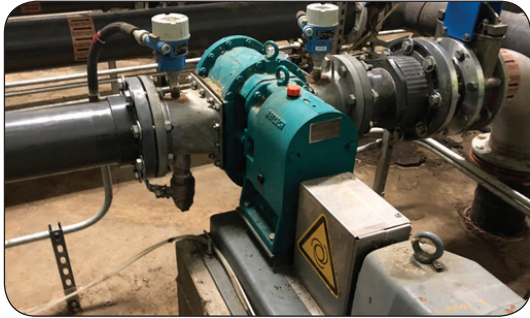
TORNADO® T1 transferring Kaolin Slurry in Paper Industry
