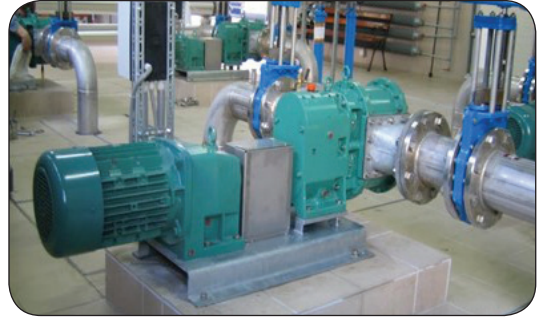
TORNADO® T1 transferring sludge in less space environment
