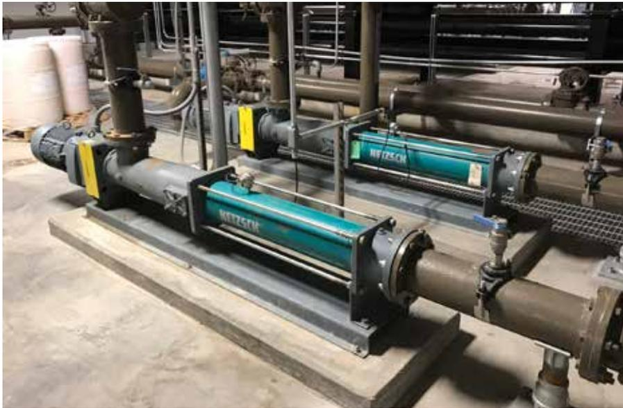
NETZSCH NEMO® 090 BY pumps in the Boiler Building transfer hydrolyzed food waste with extremely low pH product with 5% solids.
