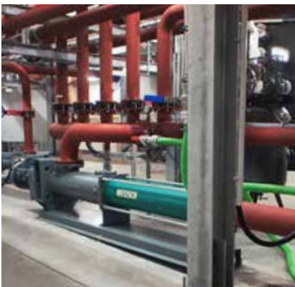
The NEMO® progressing cavity pump: an energy-efficient solution for high pressure ranges
