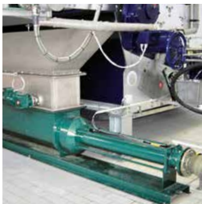
External view: NEMO® progressing cavity pump in a sewage plant with hopper and aBP-Module®
