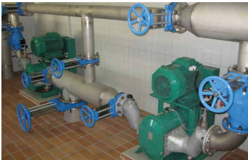
TORNADO® rotary lobe pumps for digested sludge recirculation
