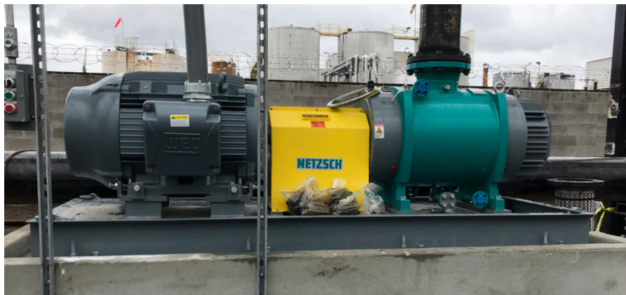
NETZSCH proposed double mechanical seals with an API 54 seal plan that provided protection from a range of viscosities.
