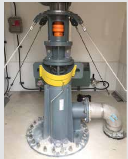
The NETZSCH BT vertical pump has reduced loading time to 17-20 minutes and while allowing increased solids content.
