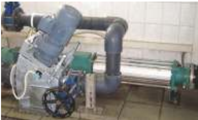
M-Ovas® macerator and NEMO® progressing cavity pump in series offers process reliability and efficiency.
