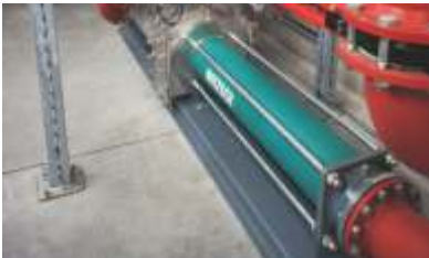
B.Max® progressing cavity pump liquid feeding for reliable and flexible substrate supply.
