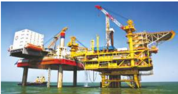
NEMO® progressing cavity pump on platform to transfer bilge oil
