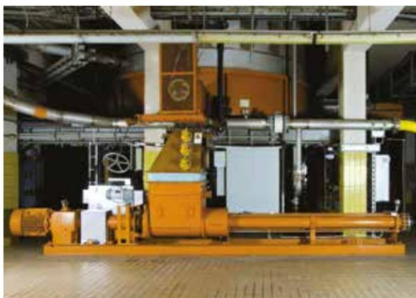
NEMO<sup>®</sup> Sludge Cake Pump with bridge breaker conveying dewatered sludge immediately overhead via a long radius elbow 270 ft. (80 m) to incinerator. Solids content approximately 25%–32%, flow-rate of 8–60 gpm (2–14 m<sup>3</sup>/hr) at 360 psi (25 bar) discharge pressure.
