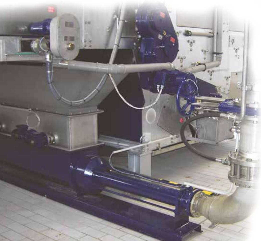
NEMO® Sludge Cake Pump with customized 4.27 ft / 1.5 m hopper pumping 20 - 22% dewatered sludge from a belt filter press to a drying plant 110 ft. (34 m) away. Pump employs dual aBP-Module® (Asynchronous Bridge Preventing Module), STP stator dry running protection system and the Friction Loss Reduction System (FLR - see page 8 and 9).
