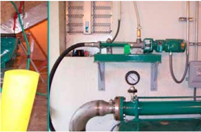
NETZSCH FLR System being used in conjunction with NEMO® Sludge Cake Pump to convey dewatered sludge over 900 ft (275 m) for transport. With the introduction of only 0.7 gpm (.16 m<sup>3</sup>/hr) of polymer into the sludge, pressures are reduced from 450 psi to 150 psi (31 bar to 10 bar) for safe and easy long distance transfer within the pipeline. Sludge cake solids content approximately 23% being pumped at 20 gpm (4.5 m<sup>3</sup>/hr).
