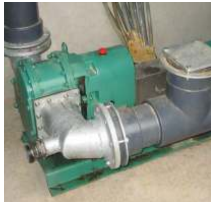
Emptying a final storage facility at a capacity of 20m 3 /h
