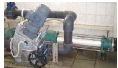
M-Ovas® and NEMO® macerator progressing cavity pump in series offers process reliability and efficiency.
