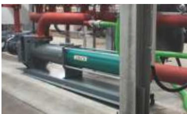
The NEMO® progressing cavity pump: an energy-efficient solution for high pressure ranges too
