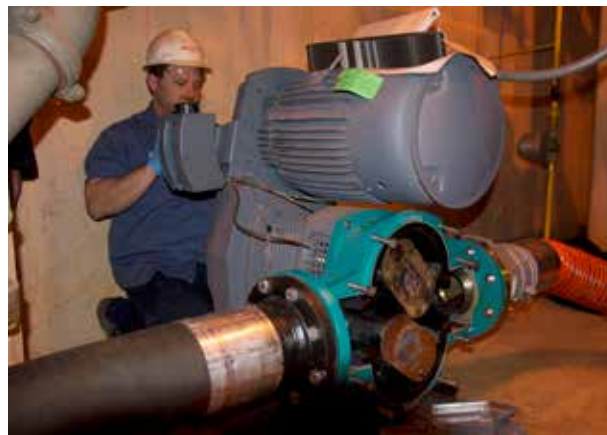
A Veolia maintenance engineer checking the NETZSCH TORNADO® T2 Rotary Lobe Pump during routine maintenance. Note the easy access to rotors from front of the pump.
