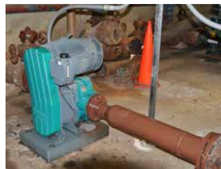
NETZSCH TORNADO® T2 Rotary Lobe Pump seen in operations in sludge transfer line.
