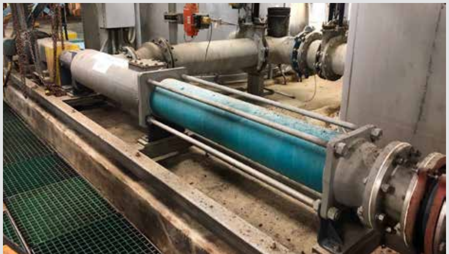
The NETZSCH NEMO® pump replaces a screw conveyor to transport the peel feed from the reaction tank to the peel press.
