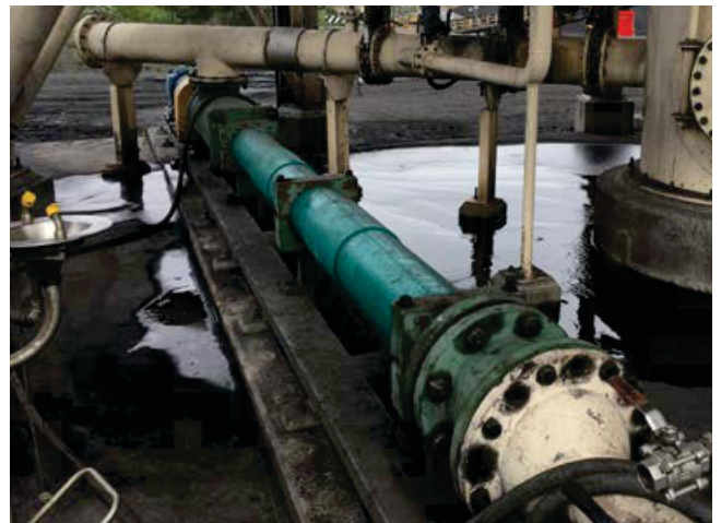
Excellent solids handling and pressure capabilities enable the handling of demanding slurries with NEMO ® progressing cavity pumps.
