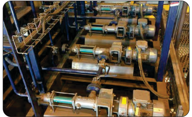
Reagent transfer using multiple NEMO® BY pumps
