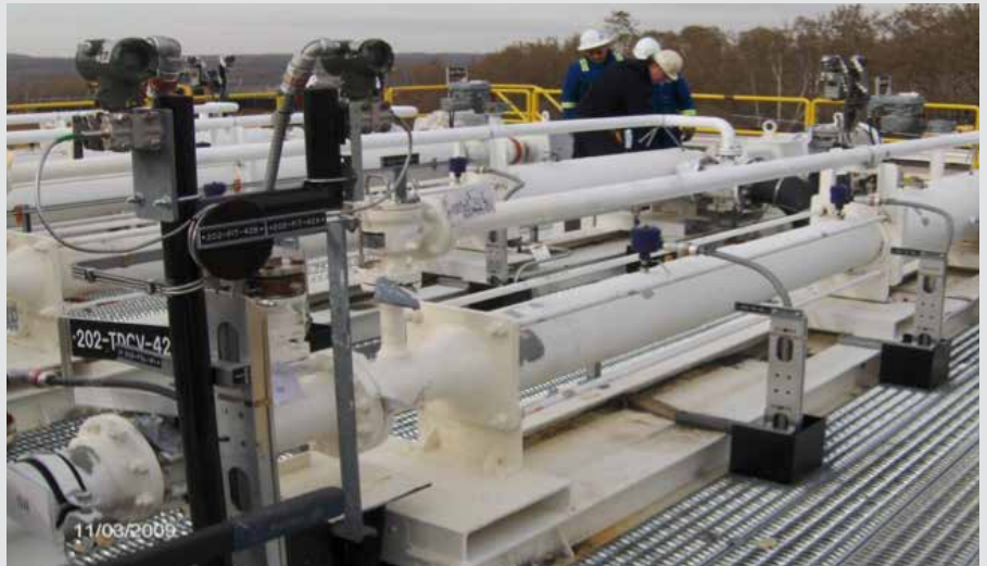
NETZSCH large progressing cavity pumps installed at customer site
