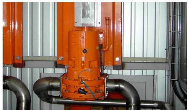
TORNADO® pump for sewage water
